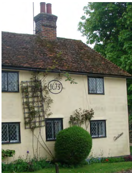
Picture 1.3 Pargetting, colour-washed plaster and simple detailing on Centuries in Church Road
