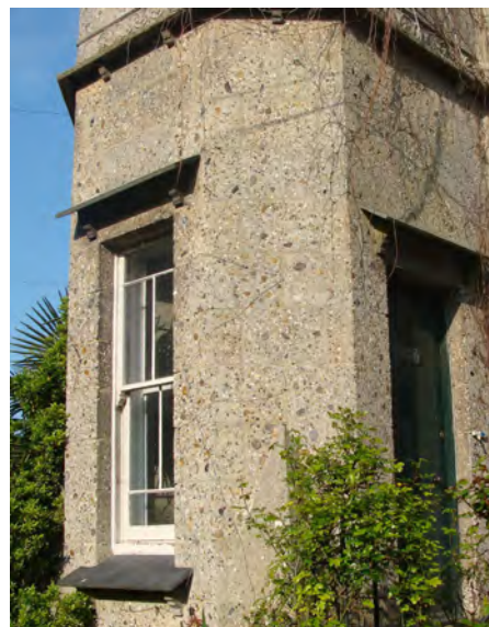
Picture 1.4 Glebe House constructed of concrete and exposed aggregate block detailing in the Scottish Baronial Style
